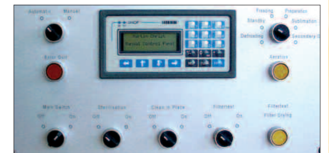
17.2.: Additional control panel with manual controls (redundant)
