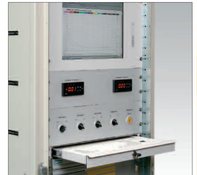
17.1.: Industrial PC with SCADA software LPC for system control
