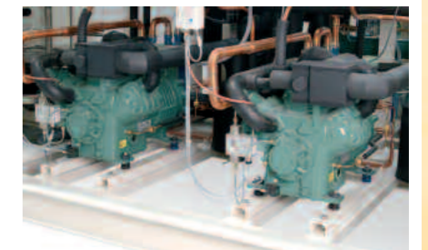
11.2.: Redundant cooling system
